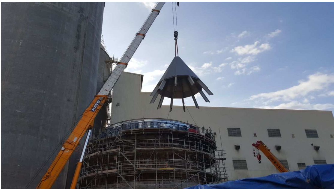
Inner cone in electro welded steel structure
